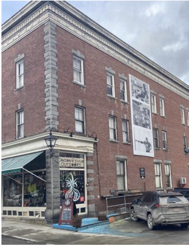
20 Langdon Street/Onion River Outdoor Building
